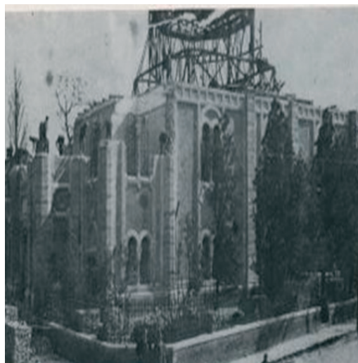
Demolition of the Zrenjanin Synagogue in 1941
